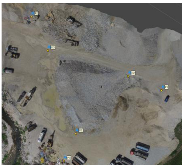
Figure 4. Geodetic Base of the Terrain
