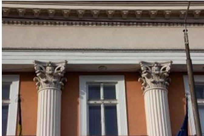
Figure 7. Corinthian columns - Deschan Palace
